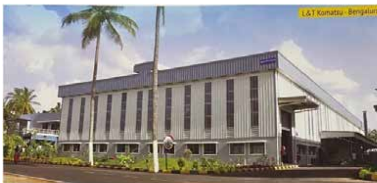
Fig. 3: L&T office building – Bengaluru [ Courtesy: PEBS Pennar ]
