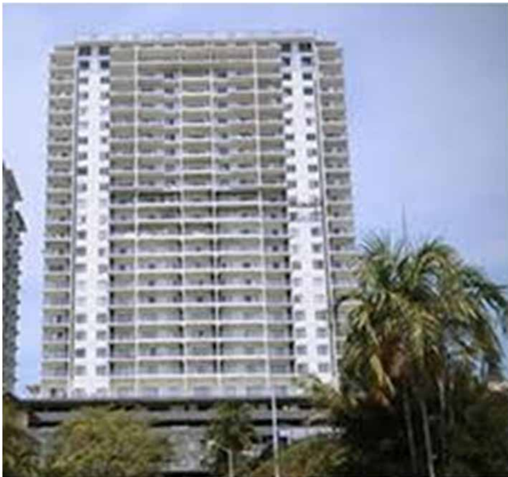
Fig. 23: Soho Apartment, Darwin, Australia [9]
