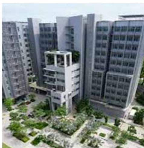
Fig. 17: NTU North Hill Hostel [11]
