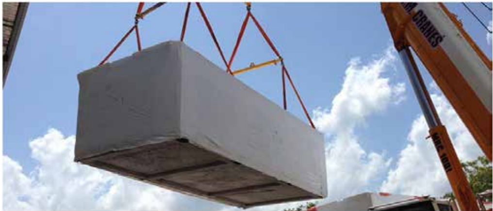
Fig.22: Lifting of Unit [13]
