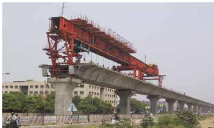
Fig 2: Viaduct Installation [ Courtesy DMRC ]
