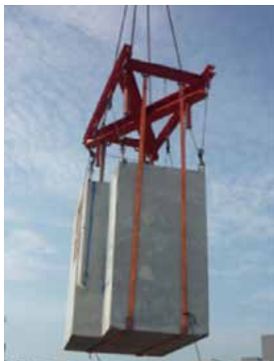
Fig. 13: Lifting PBU in Place [7,8]
