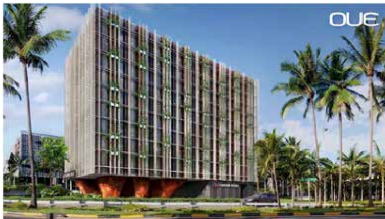
Fig. 18: Crowne Plaza Hotel Extension [12]
